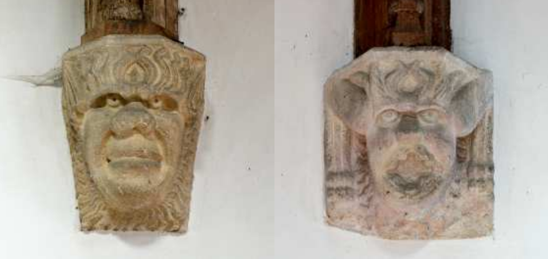
Two of the corbels at Lyddington. Photographs by Mike Walter.
